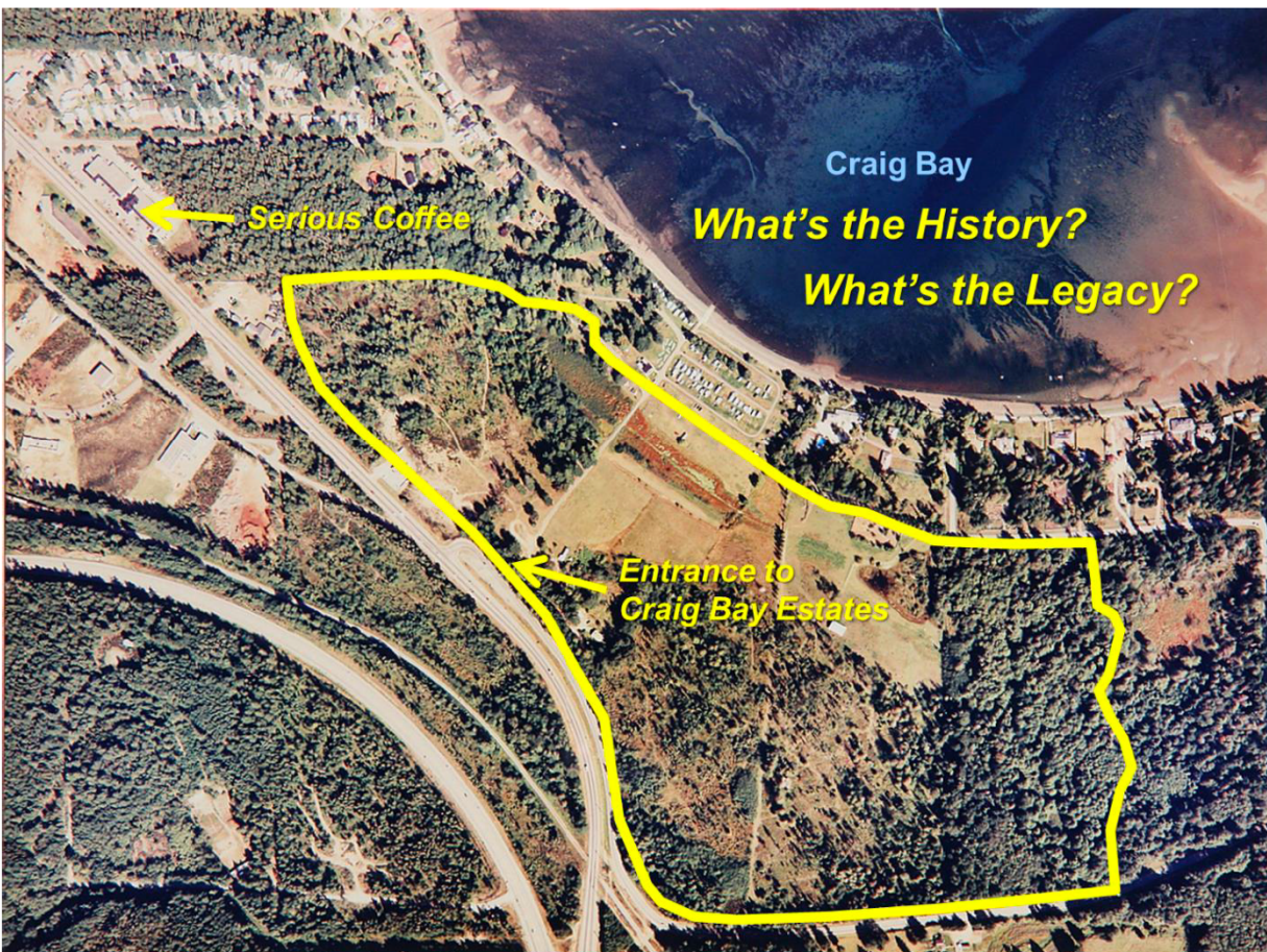
Fig. 2: Aerial photo of the lands within which CBE (yellow outline) was later developed.
