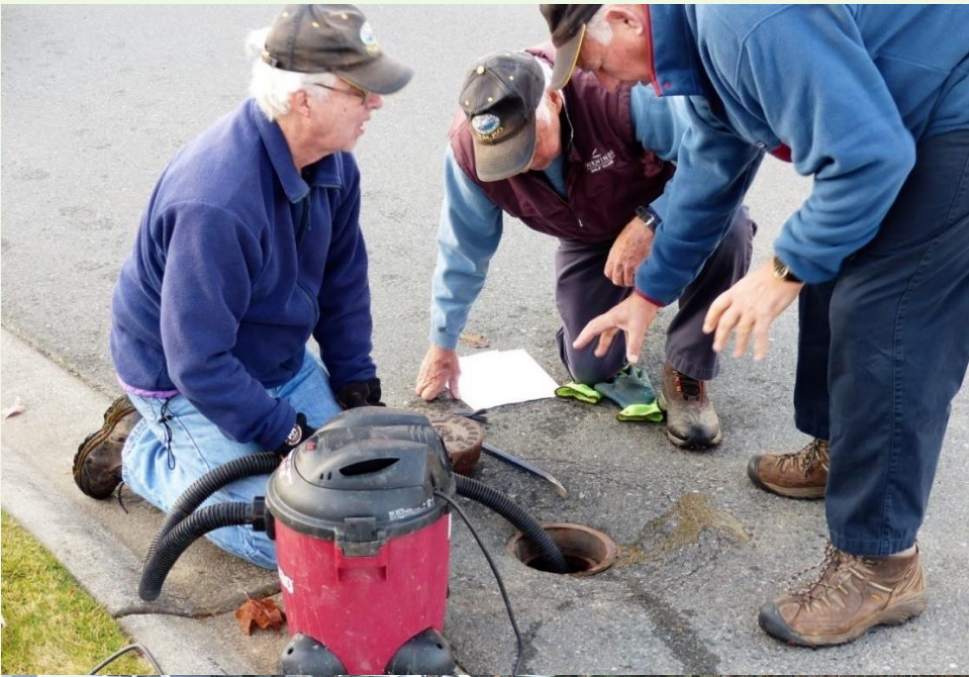
Keeping close tabs on Craig Bay's vast underground systems.
