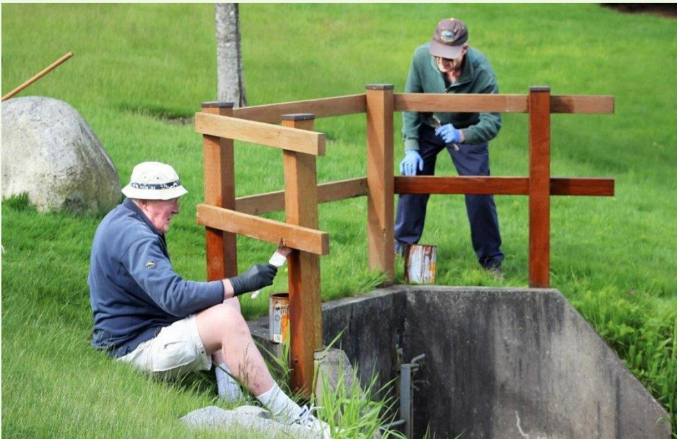
Giving safety fences, foot bridges and signposts fresh coats.
